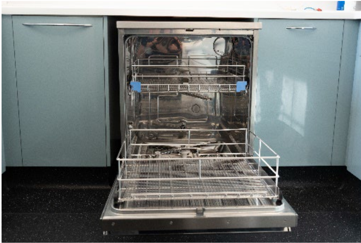
Figure 2.3 - Under bench washer disinfector shown with open door
