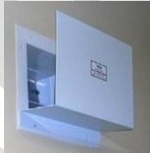
Figure 2 Pressure stabiliser fitted in preparation “lay up” room with stand-off baffle in theatre
