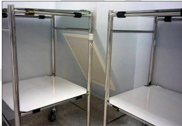
Figure A27 Low level extract recommended installation
