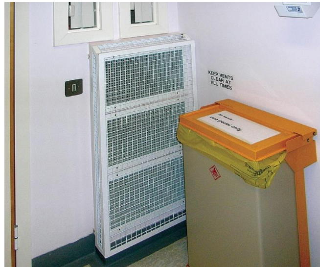
Figure 8 Pressure stabiliser with stand-off cage
