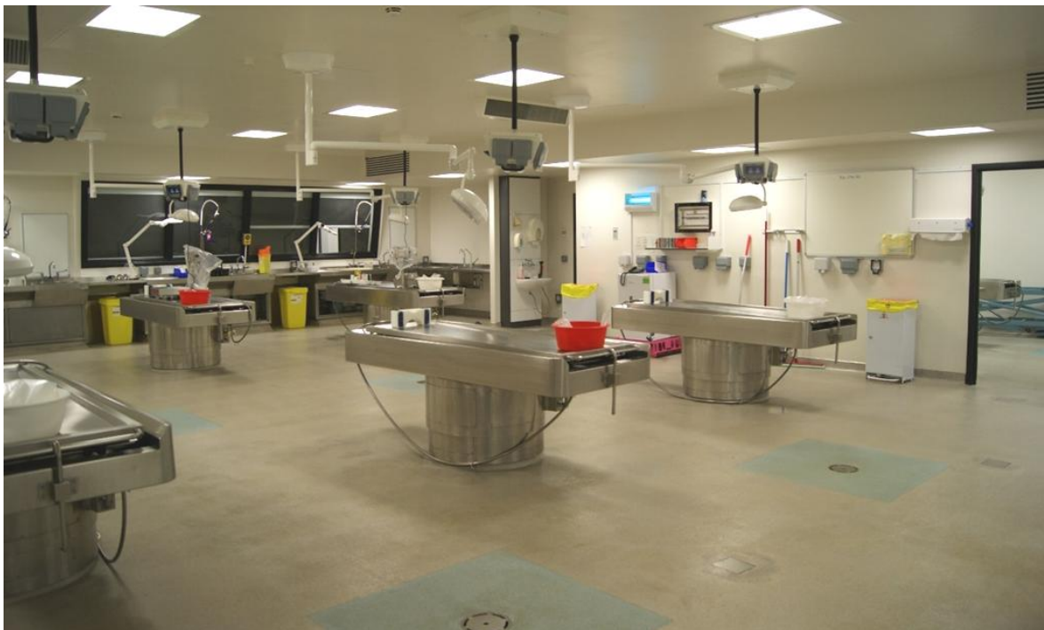
Figure 5-4: PM 6-table suite with observation room at rear, QEUH Glasgow
